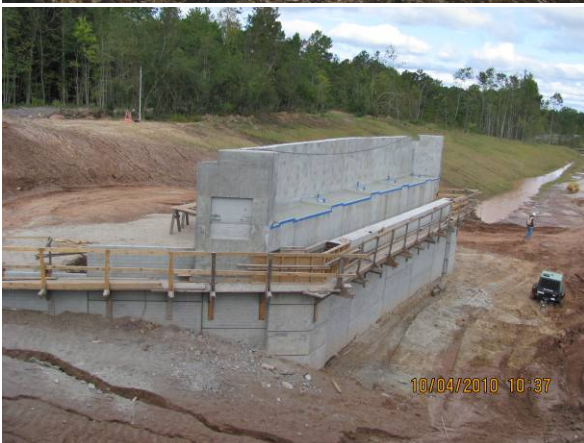
Picture 1: Site #14 US 64 – Installing MSE Panel and Backfill at End Bent #1.
