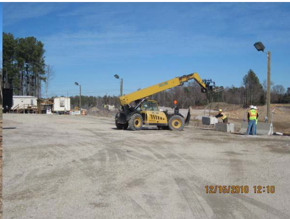
Picture 2: Grading Construction Entrance at Apex BBQ Rd Picture 4: Setting Blocks for Material Storage Bins at Batch Plant Site
