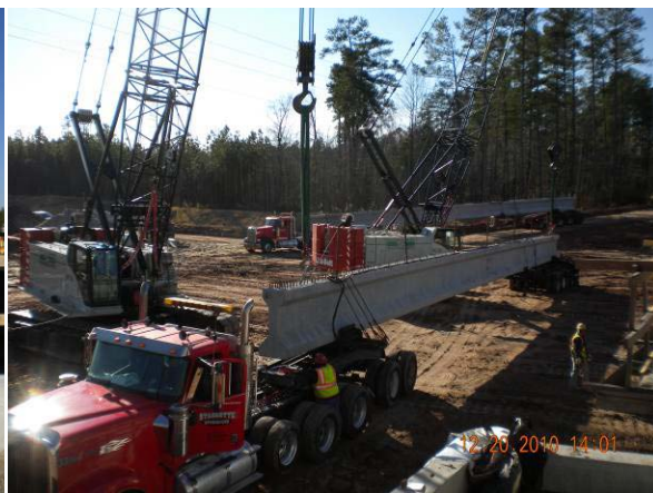
Picture 2: Site #14 US 64 -Installing ABC under approach slab End Bent NB
