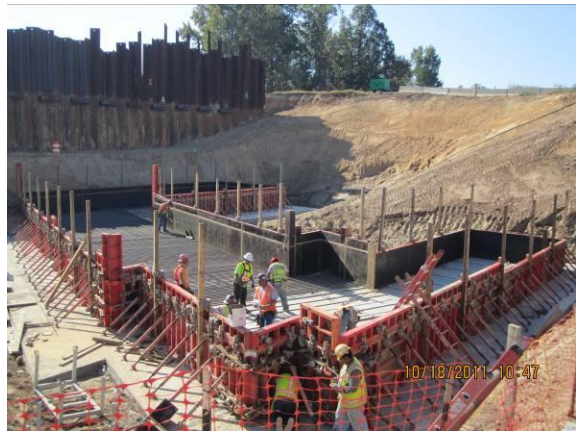
CSX – Installing rebar at EB 1 Footing
