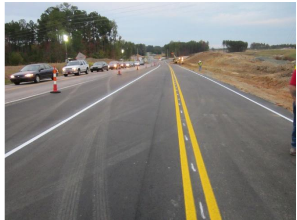
Striping Kelly Rd for Traffic Switch
