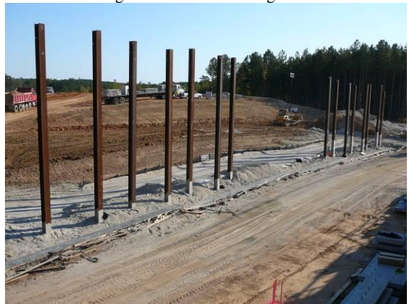
Flyover Rd – MSE Leveling Pad Poured at EB 1
