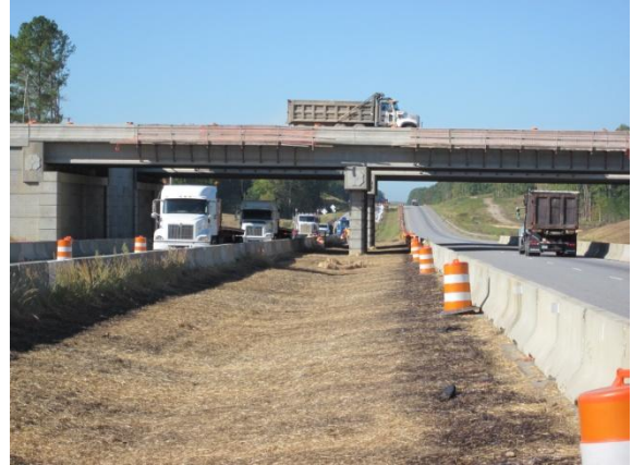
Completed Median Grading US1
