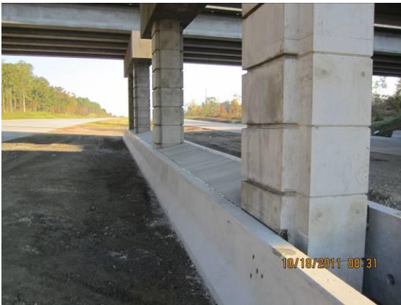
McCrimmon – Precast Barrier Backfilled and Capped.
