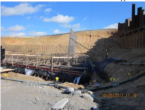
CSX – Installing cooling tubes at EB 2 Footing
