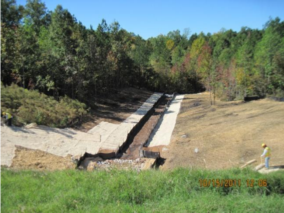
Area Graded after Sediment Basin Removal
