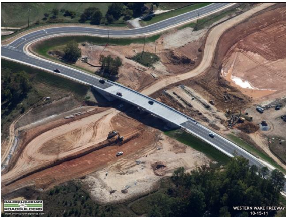
Mass Excavation North and South of Jenks Rd
