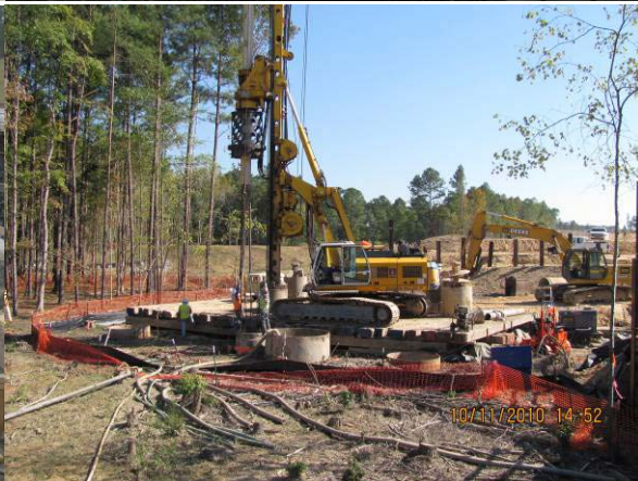
Picture 2: Site #26 Nancy Branch – Pouring SB Bridge Deck Picture 4: Site #11 Beaver Creek – Coastal Caisson drilling shafts Bent #1 NB
