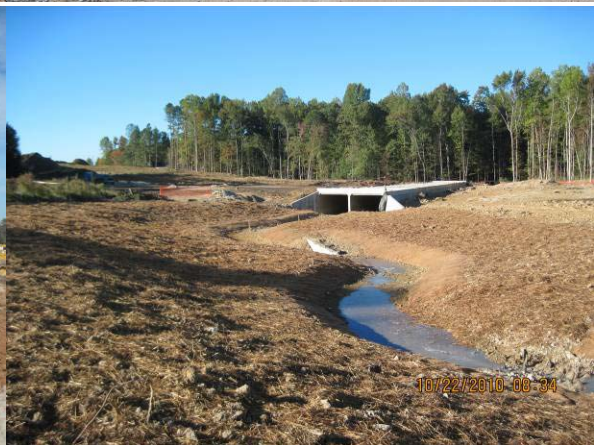
Picture 2: Placing ABC Stone at Ramp C of Hwy 55 Interchange Picture 4: Stream Relocation Into Box 9 South of US 64
