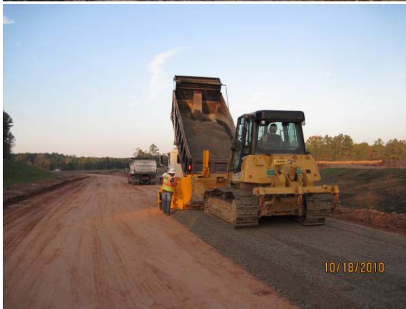
Picture 1: Chemical Stabilization South of Carpenter Fire Picture 3: Placing ABC Stone at Hwy 55 Ramp
