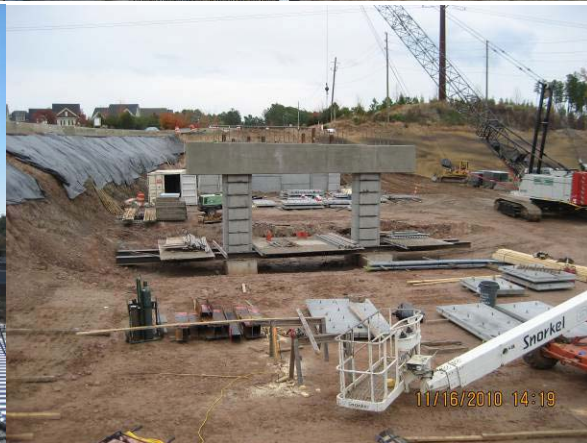
Picture 2: Site #26 Nancy Branch- Forming End Bent #2 SB approach slab Picture 4: Site #24 RT Carpenter Fire Station Rd – Stripped cap
