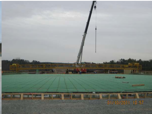
Picture 2: Site #19 White Oak Creek – Pumping Span D NB Deck Picture 4: Site #14 US 64 – Bidwell setup for deck pour
