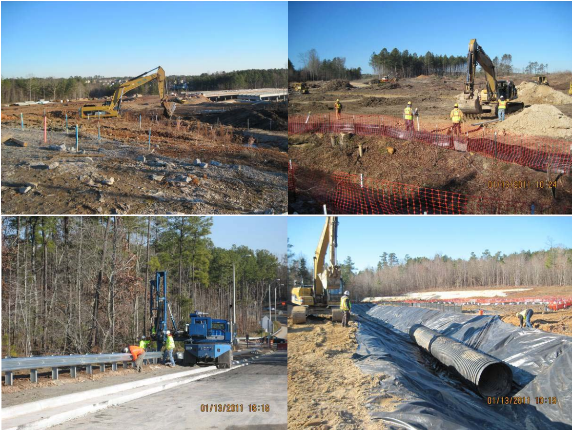
Picture 1: Constructing Basins for Batch Plant Site
