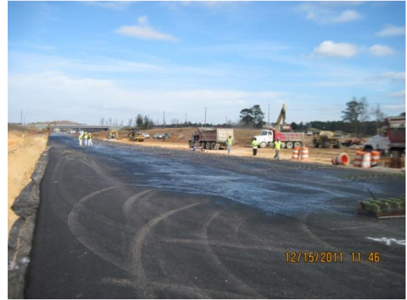
Set up for Concrete Paving North of US 64 (C2)
