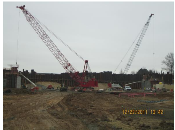
Site #8 CSX Railroad – Stripping forms and forming backwall
