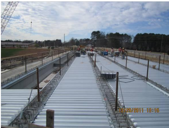
Site #12 Olive Chapel Rd – Installing SIP decking
