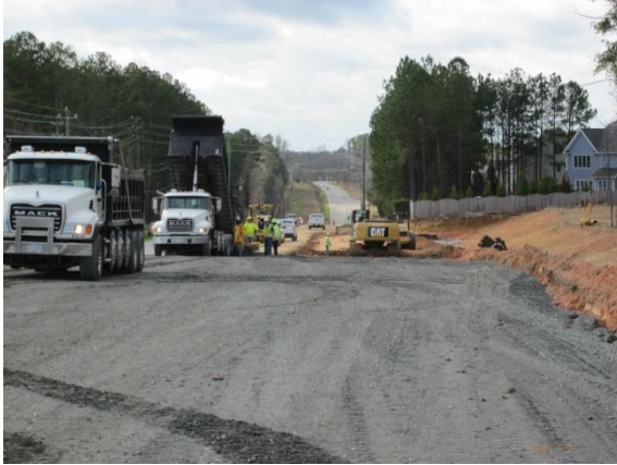
Grading New Alignment at Kelly Rd
