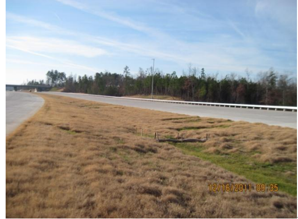
Guardrail South of McCrimmon Parkway (C11)
