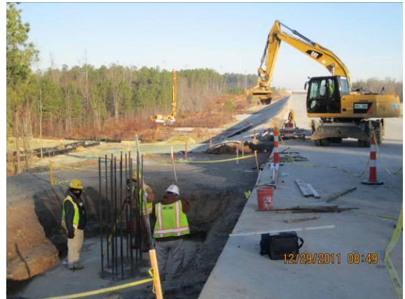
ORT Site #5 – Excavating gantry foundations
