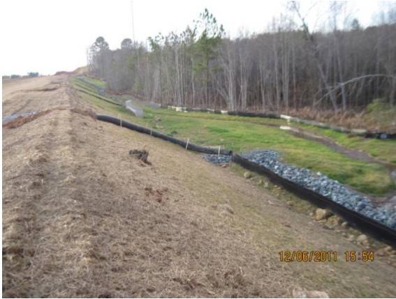
Phases of Seeding on fill Slopes North of Hwy 55 (A2)
