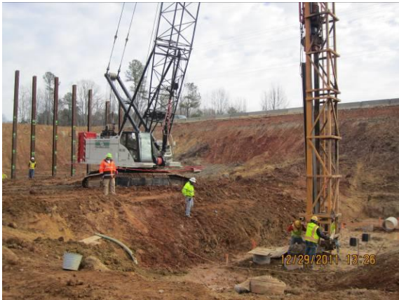
Site #10 Apex Barbeque Rd – Driving pile at Bent #1
