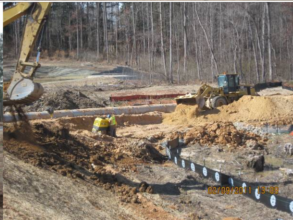
Picture 2: Chipping Clearing Debris South of US 1
