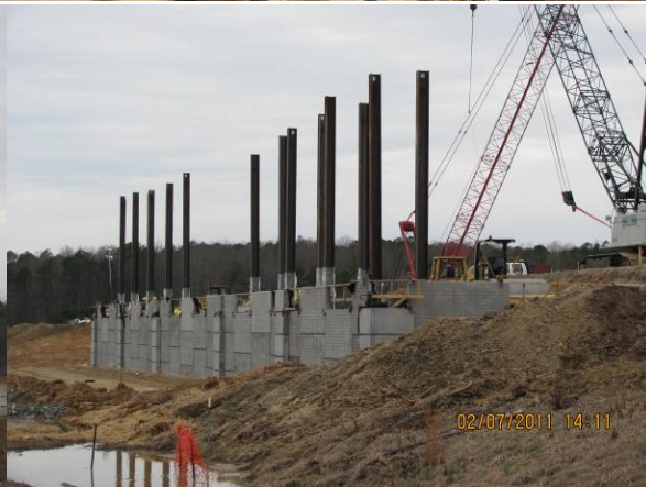
Picture 2: Site #24 Carpenter Fire Station Rd (RT) – Pouring bridge deck Picture 4: Site #6 US 1 – Install MSE Panels
