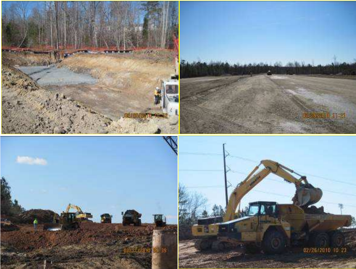
Picture 1: Excavation at Box Culvert 15 Picture 3: Clearing south of Nancy Branch
