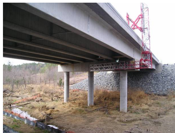
Panther Creek – Striping South Bound Diaphragms
