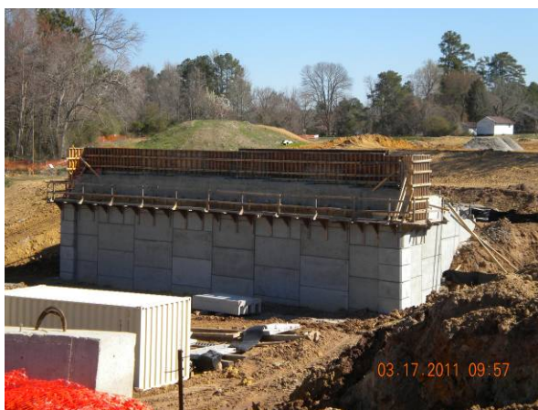
Green Level West – Forming End Bent Backwall
