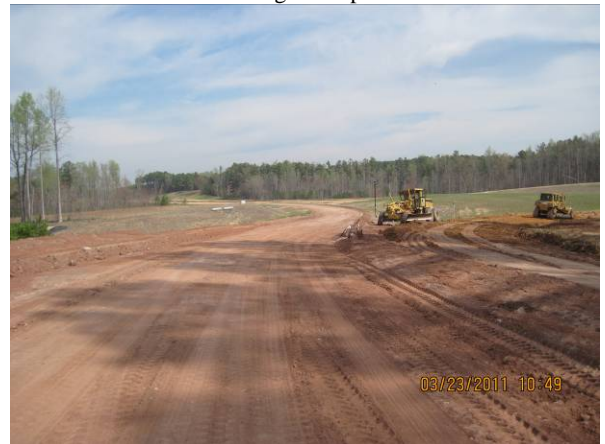
Finegrading Ramps at Green Level West
