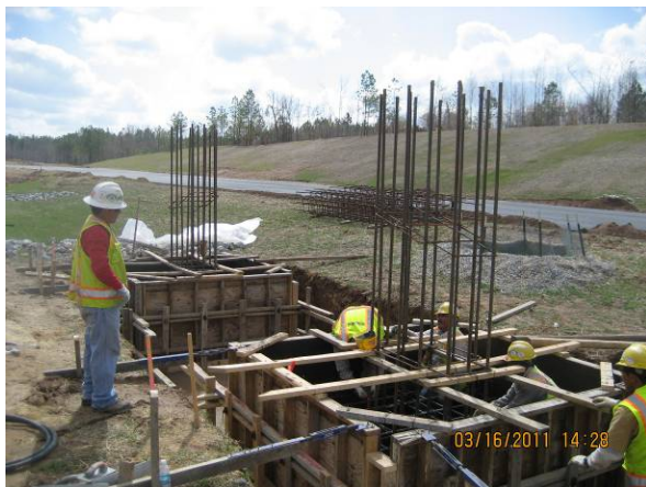
Morrisville Parkway-Forming Bent Footings
