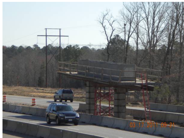
Flyover Bridge – Striping Bent Cap
