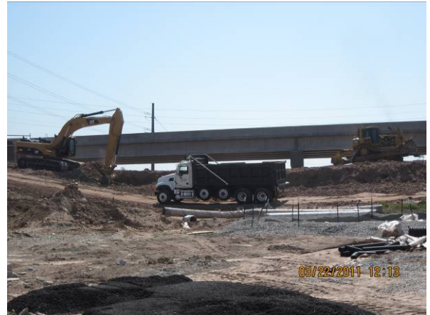
Excavation of Mainline Plug at Carpenter Firestation
