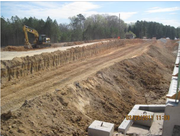
Excavation of Roberts Rd
