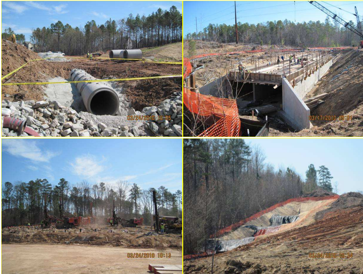
Picture 1: 60in RCP Between Carpenter Fire and Panther Creek Picture 3: Drilling for Mass Blasting North at Panther Creek
