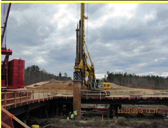
Picture 1: TWC Installing OH Lines on temp poles at Carpenter Fire Station Picture 3: Installation of Drilled Shafts @ Site #23 – Panther Creek
