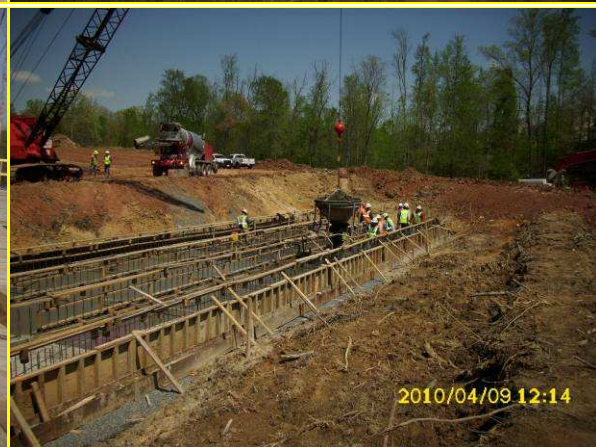
Picture 2: Finished Slope South of Nancy Branch Picture 4: Placing Concrete Box Culvert 14
