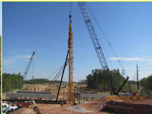
Picture 2: Assembling Temporary Trestle Bridge @ Site 19 Picture 4: Driving permanent H-Pile @ Site 26 Nancy Branch
