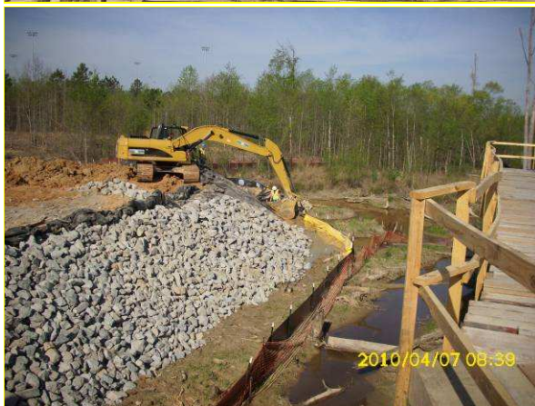
Picture 1: Drilling & Blasting Crew North of Panther Creek Picture 3: Installing Erosion Protection adjacent to Panther Creek
