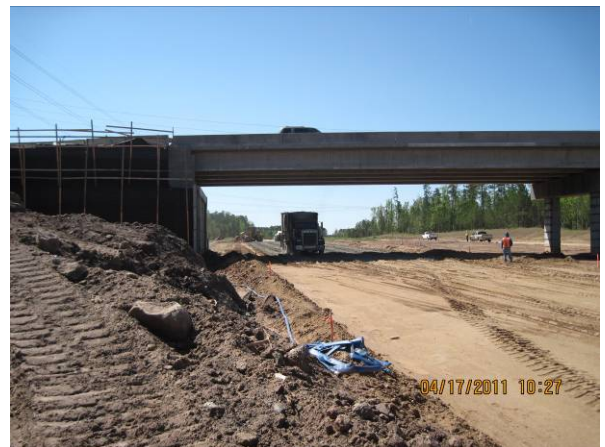
Soil Stabilization at Carpenter Fire Station Main Line Plug
