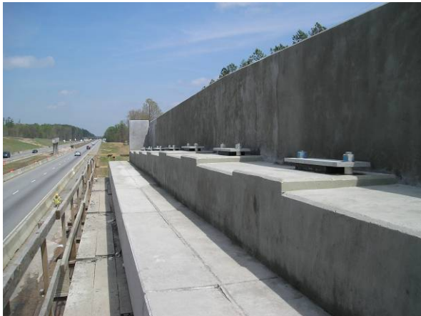
End Bent #1 NB beam seats prepped for girders
