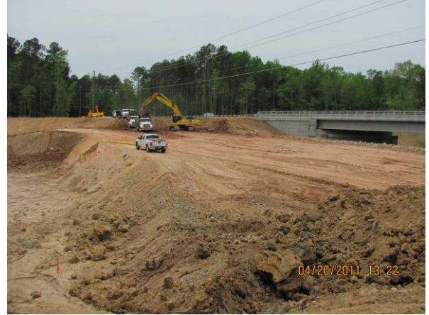
Excavation of Green Hope School Plug
