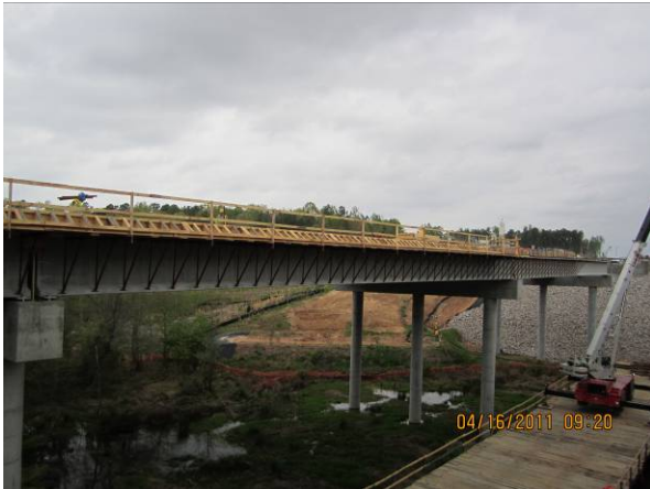
White Oak Creek – Installing OH jacks on SB bridge
