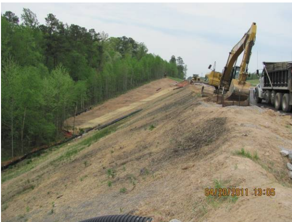
Rough Grading Shoulders North of Green Hope
