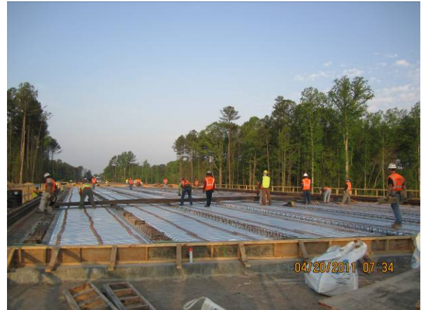
Green Level West – Installing deck rebar
