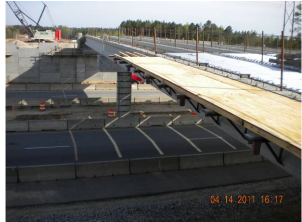
Installing OH jacks on SB bridge
