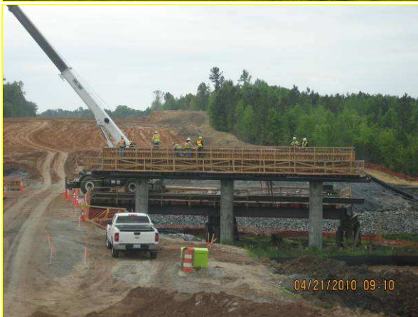
Picture 1: Setting Precast Girders at Site #26
