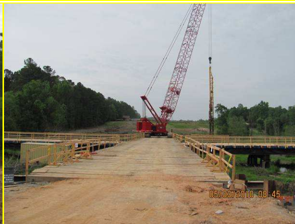
Picture 2: Drove Pile for Bent 1 SB & NB at Site 25 Picture 4: Completed Trestle Bridge at Site 19
