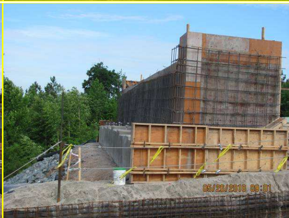
Picture 2: Site #14 Started Pre Auger & Drive Pile at Bent #1 Picture 4: Site #23 Pour and Strip End Bent #2
