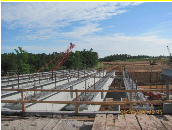
Picture 1: Site #25 Form Aesthetic Cap at Bent #1 Picture 3: Site #26 Erect Girders Span A Girders
