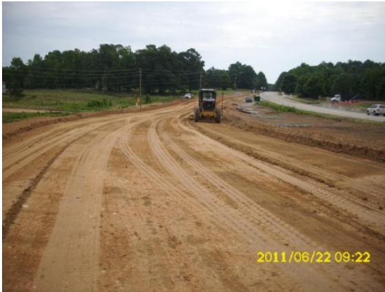
Fine Grading Olive Chapel Detour
