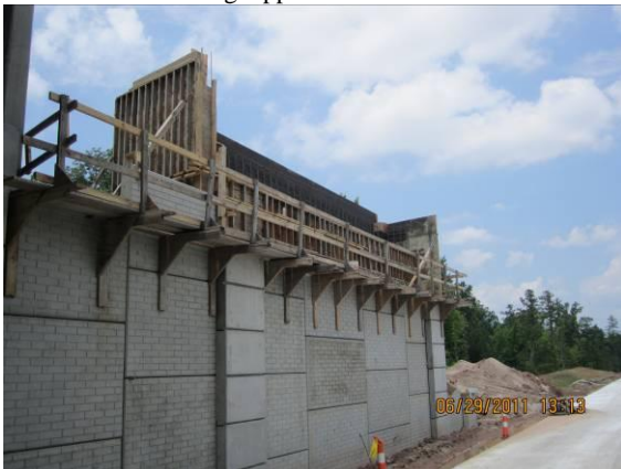
Site #24 Carpenter Fire Station – Forming EB1
