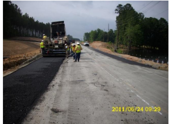
Paving Kelly Rd Widening
