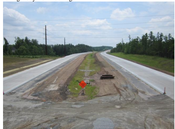
Concrete Paving South of Carpenter Fire Station
