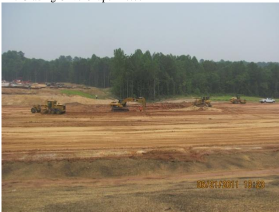
Undercut, Backfill and fine grading South of Green Level West
