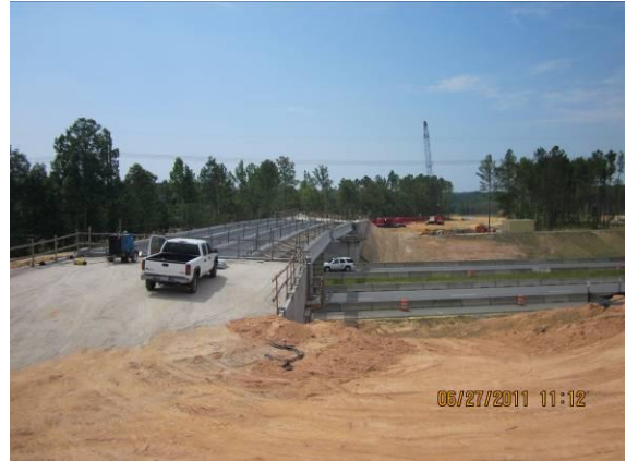
Site #7 Flyover Bd – Girder Set
