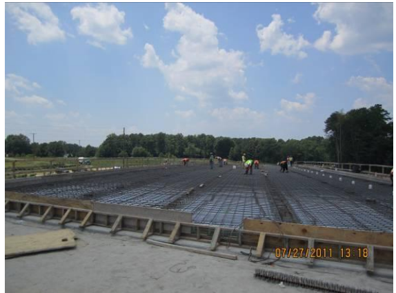
Site #16 Jenks Rd -Tying Deck Steel
