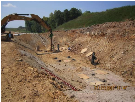
Site #13 Beaver Creek - Preauger Pile at End Bent #1
