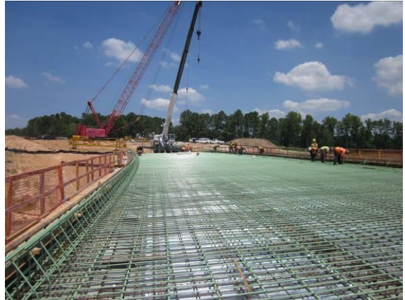
Site #7 Old US1– Prepping Deck Steel
