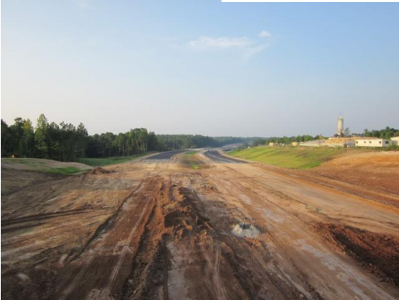
Fine Grade Stabilization South of Green Level West
