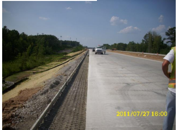
Forming Shoulder Berm Gutter North of Green Level West
