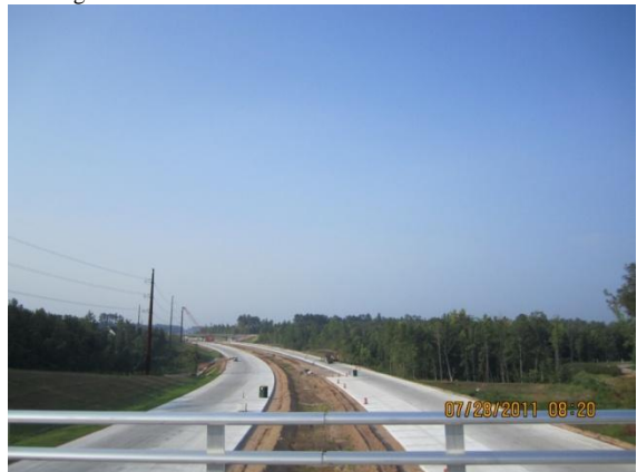
PCCP as seen on McCrimmon Pkwy facing South
