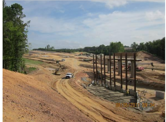
Site 13 Beaver Creek Commons EB1 North
