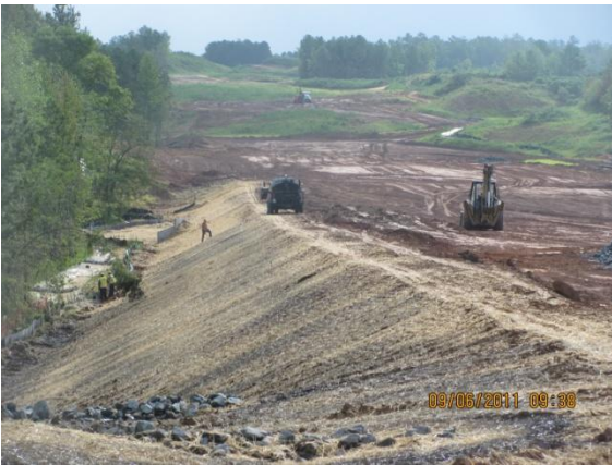
Seeding Fill Slope in
