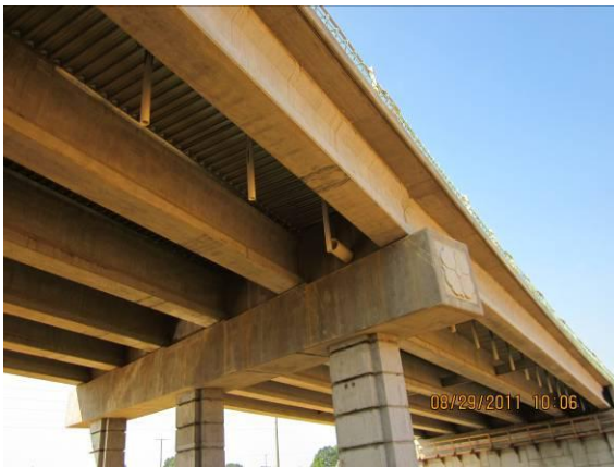
Site 16 Jenks Rd Deck Drainage
