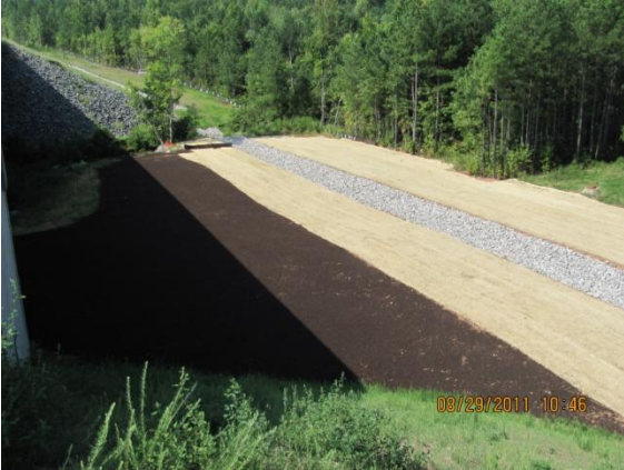
Lateral Ditch after Basin Removal Complete
