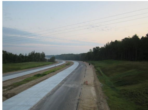
Concrete Paving North of Roberts Rd
