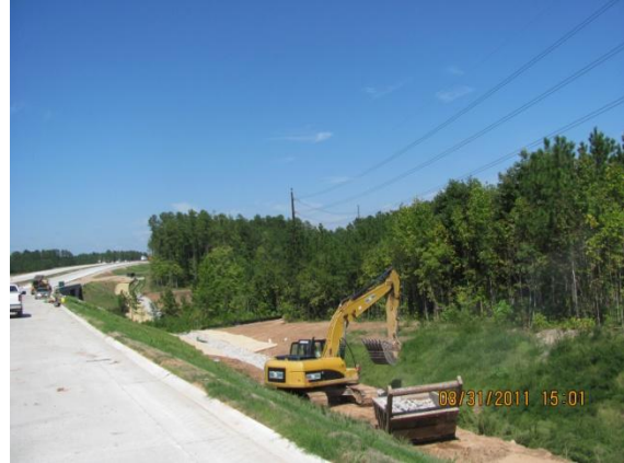
Placing Rip Rap in Lateral Ditch
