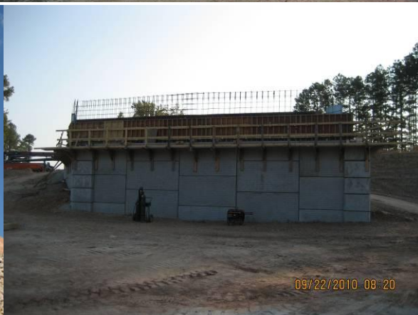
Picture 2: Site #14 US 64- Forming Bent #1 NB Cap Picture 4: Site #21 Green Hope School –Form End Bent #2
