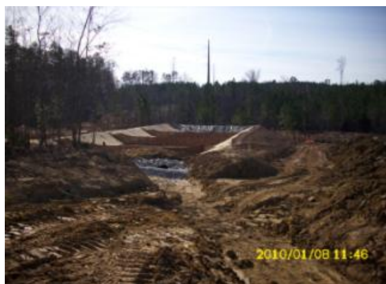
Picture 1: RDR Installing Sediment Basins at CFS Road Picture 3: Type B sediment dam at south of CFS Road
