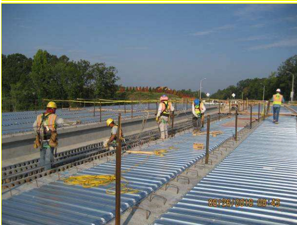
Picture 1: Site #14 US 64 Forming SB Bent #1 Cap
